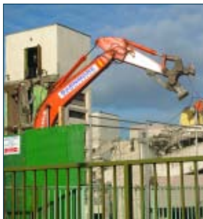
Demolition continues in preparation for the new development Photo: Denis Geoghegan
